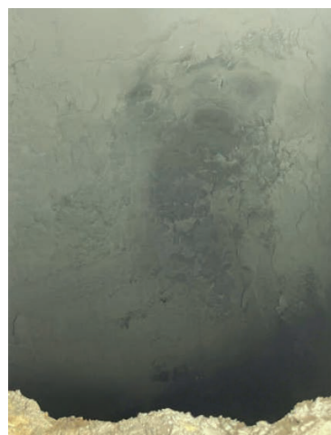
Fig. 20 Photo of repaired part.
