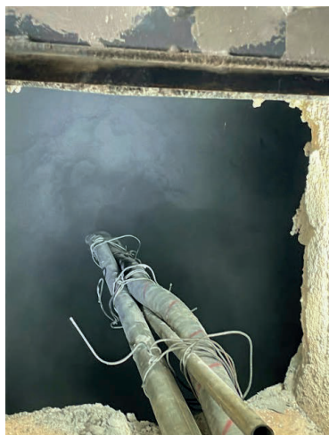
Fig. 19 Photo of gunning process.
