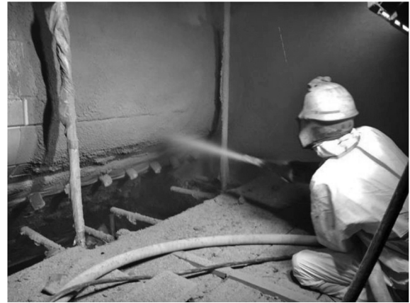
Fig. 11 Photograph of dry gunning operation in practical application.
