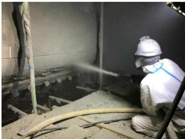
Figure 11 Appearance of gunning Material A
