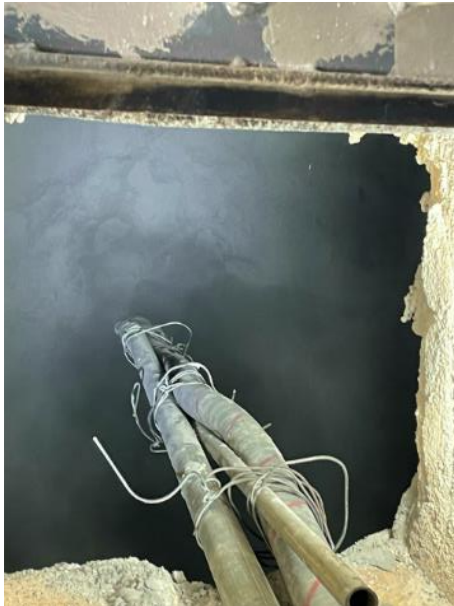
Figure 14 Appearance of gunning in hot condition
