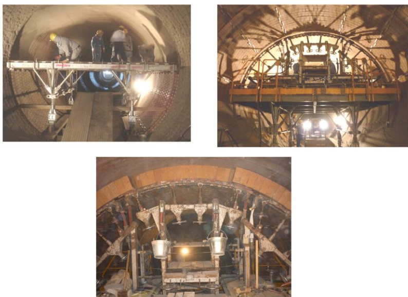
Fig. 3 The view of refractory construction using line-chess.
