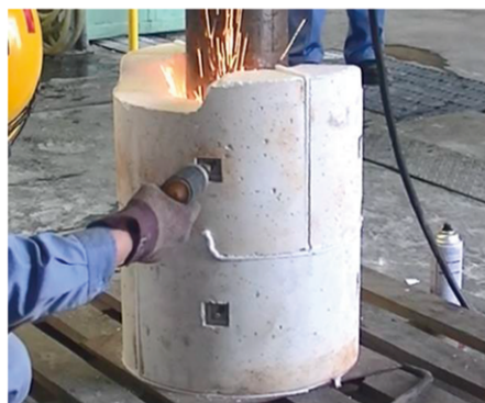
Fig. 3 Appearance of Stud gun Welding
