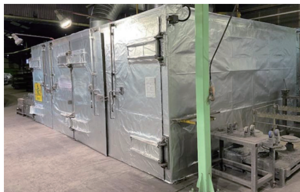
Photo 5-1 Drying furnace with heat shield sheets
