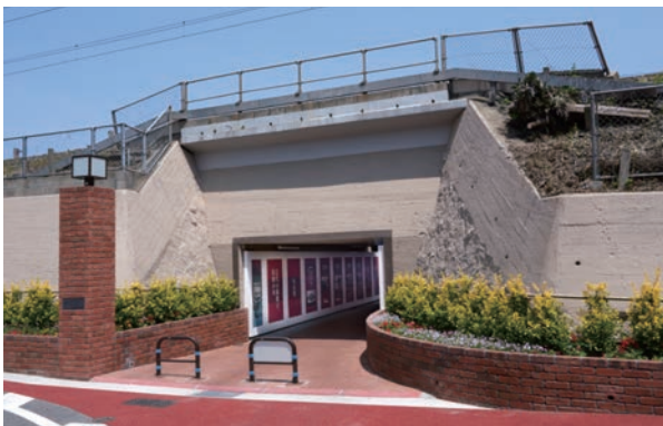
Photo 6-6 Higashihamamachi Route 1 Railway Underpass
