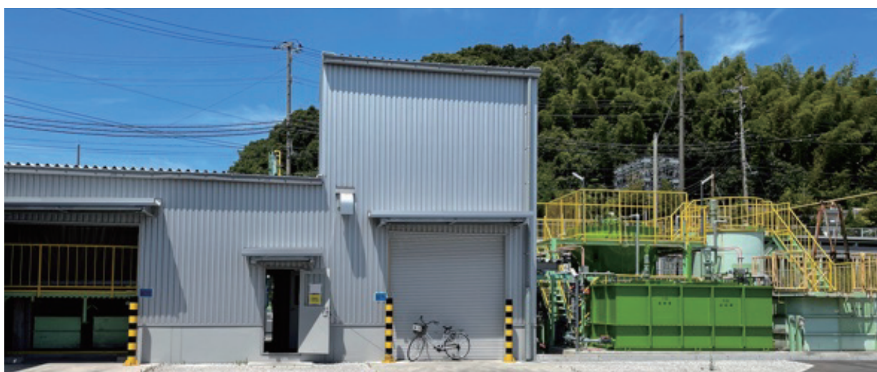
Photo 5-6 Water treatment facility (Yahata Area)
