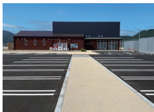
Photo 5-14 Sone Rinkai Park (Kokura-Minami Ward)
