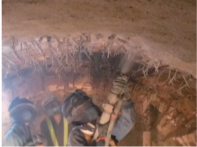
Fig. 1 Wet gunning to ceiling application with Activator F2
