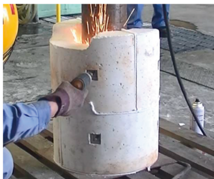
Fig. 3 Appearance of Stud gun Welding
