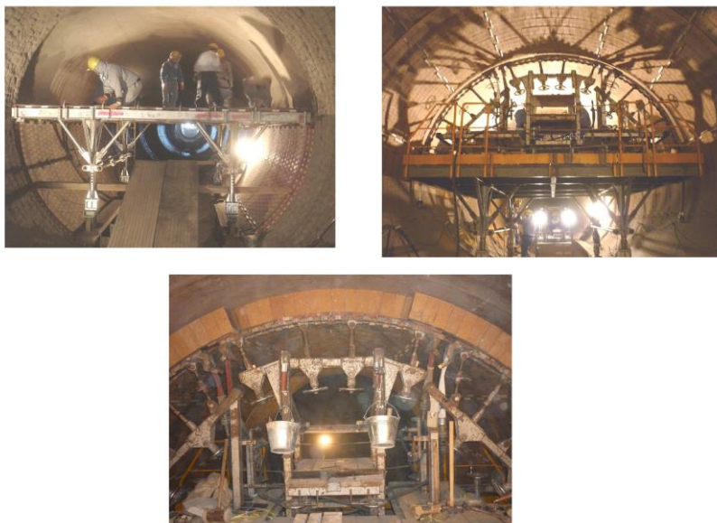
Fig. 3 The view of refractory construction using line-chess.
