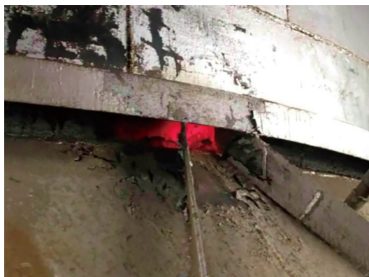
Fig. 17 Photo of steel shell red-hot part.
