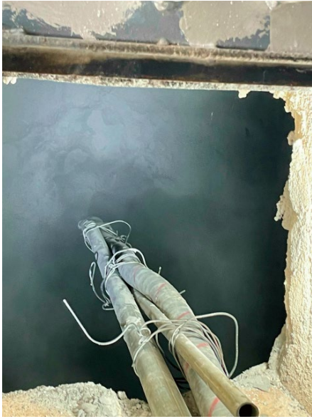
Fig. 19 Photo of gunning process.
