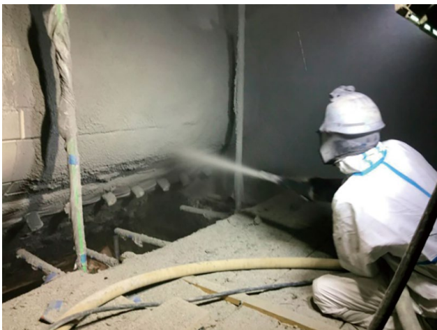
Fig. 15 Photo of actual furnace construction.
