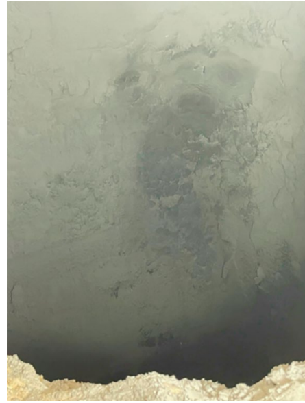
Fig. 20 Photo of repaired part.
