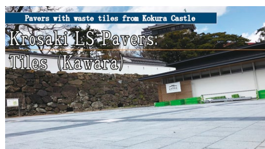
Pavers with waste tiles from Kokura Castle Krosaki LS Pavers: Tiles (Kawara)
