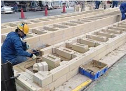
Refractories work in a coke oven
