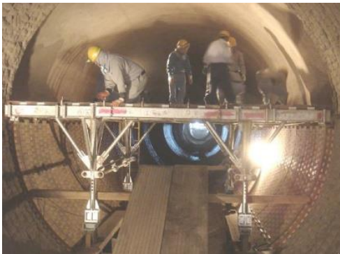
Refractories work inside a rotary cement kiln
