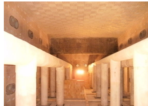
Refractories work inside a heating furnace
