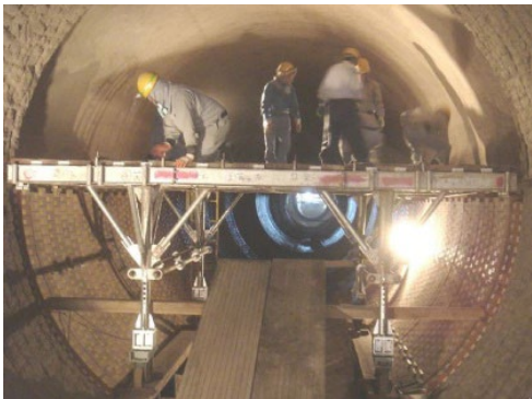
Refractories work inside a rotary cement kiln
