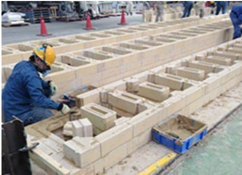
Refractories work in a coke oven
