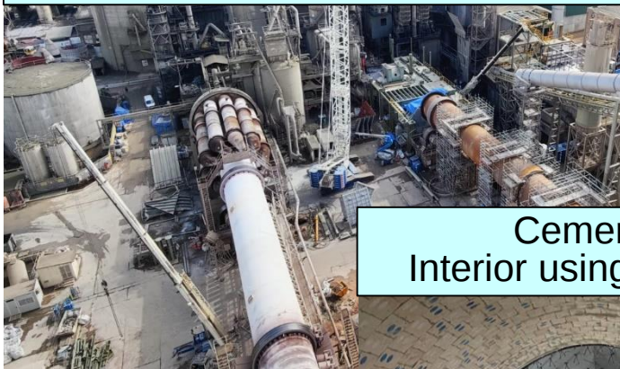
Cement kiln: Exterior
