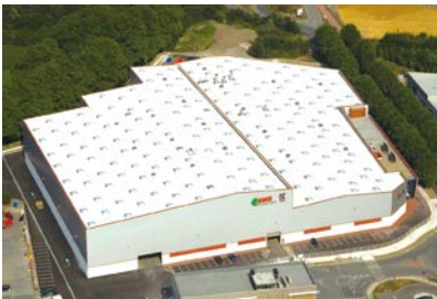
Krosaki Amr Refractories, S.A. new plant A new factory was built in Europe to strengthen the global manufacturing bases
