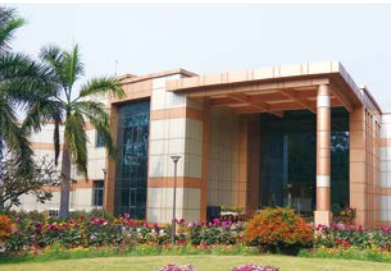
TRL KROSAKI REFRACTORIES LIMITED TATA REFRACTORIES LIMITED (now TRL KROSAKI REFRACTORIES LIMITED), the largest refractories company in India, was acquired as a subsidiary with the aim of expanding sales in India and other Asian countries
