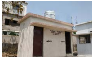
Toilet installation for local hygiene improvement and better town development
