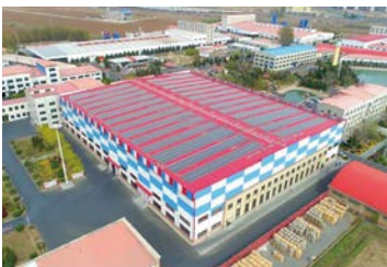
YKR's new No. 2 plant
