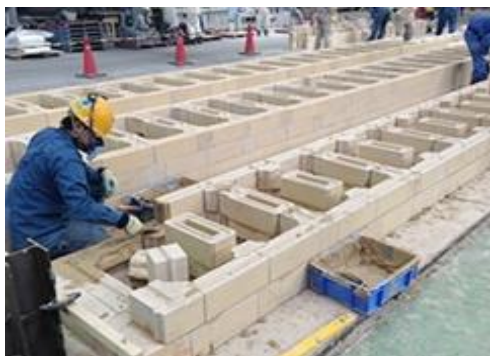
Refractories work in a coke oven
