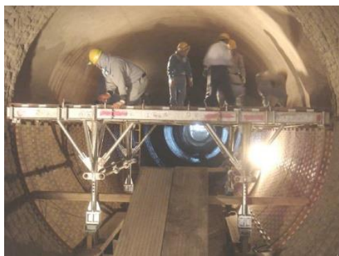
Refractories work inside a rotary cement kiln
