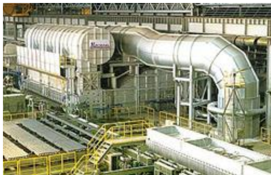
Example of construction work: pusher type billet continuous hot rolling heating furnace
