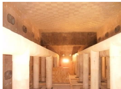
Refractories work inside a heating furnace
