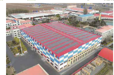
YKR's new automation plant
