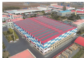
YKR's new automation plant
