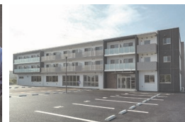
Nakano Dormitory (Kimitsu City, Chiba Prefecture) Completed in March 2023
