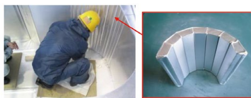
Installing insulation in a metal (iron, aluminum) melting furnace
