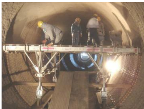
Refractories work inside a rotary cement kiln
