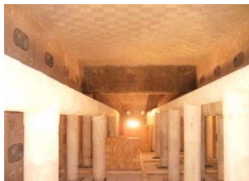
Refractories work inside a heating furnace
