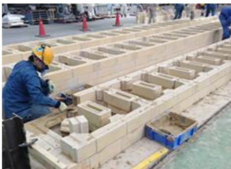
Refractories work in a coke oven
